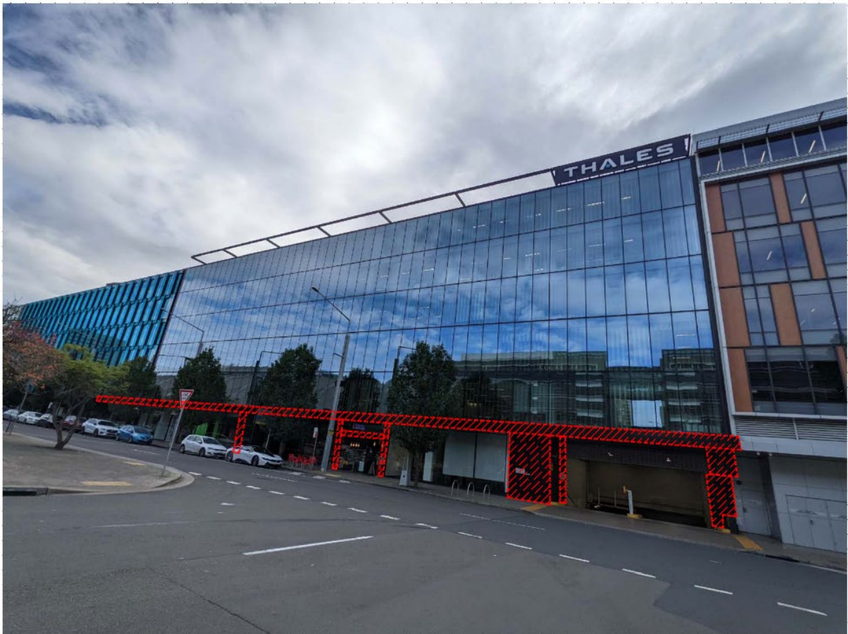
Figure 2 Photo of Southern Façade Showing Location of Cladding to be Replaced
